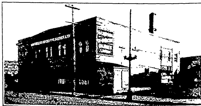
THE BRANDON PLANT OF MANITOBA CO-OP. DAIRIES.
